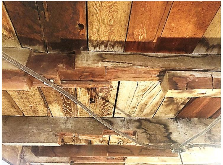
*A notched joist above the shop floor made to accommodate a belt and machine no longer in the Mill. Metal clad wiring later secured within the notch suggests the notch pre-dates 1920 when the Mill first received electric service.*
